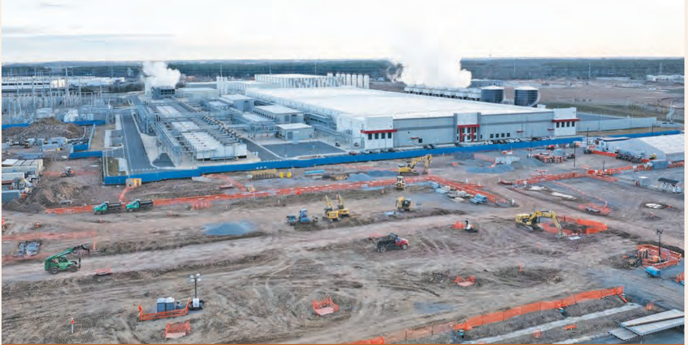
This data center was recently built in northern Virginia, host to a large concentration of data centers.
