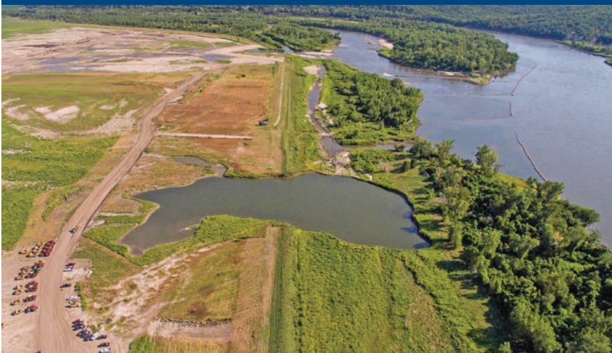
Construction of a new levee setback near a breach of the old levee.
